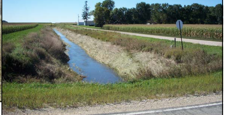
CD #6 - Open Ditch Showing High Water Line
