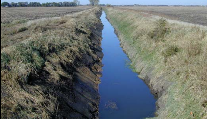
CD #5 - Open Ditch with Grass Buffers
